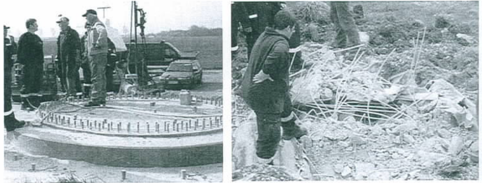
Figure 9 left: Foundation with steel ring, right: blasting result
